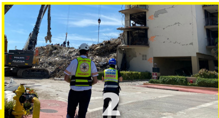
Miami Disaster Scene: "Work Around the Clock Professionally and Carefully under Complex Conditions"
